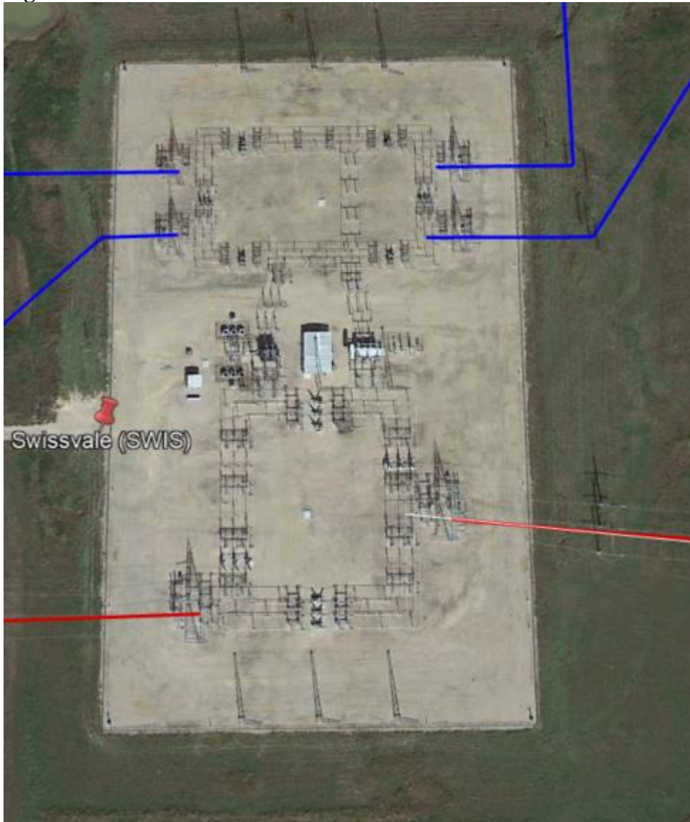
Figure 25 – Swissvale 345kV Substation
