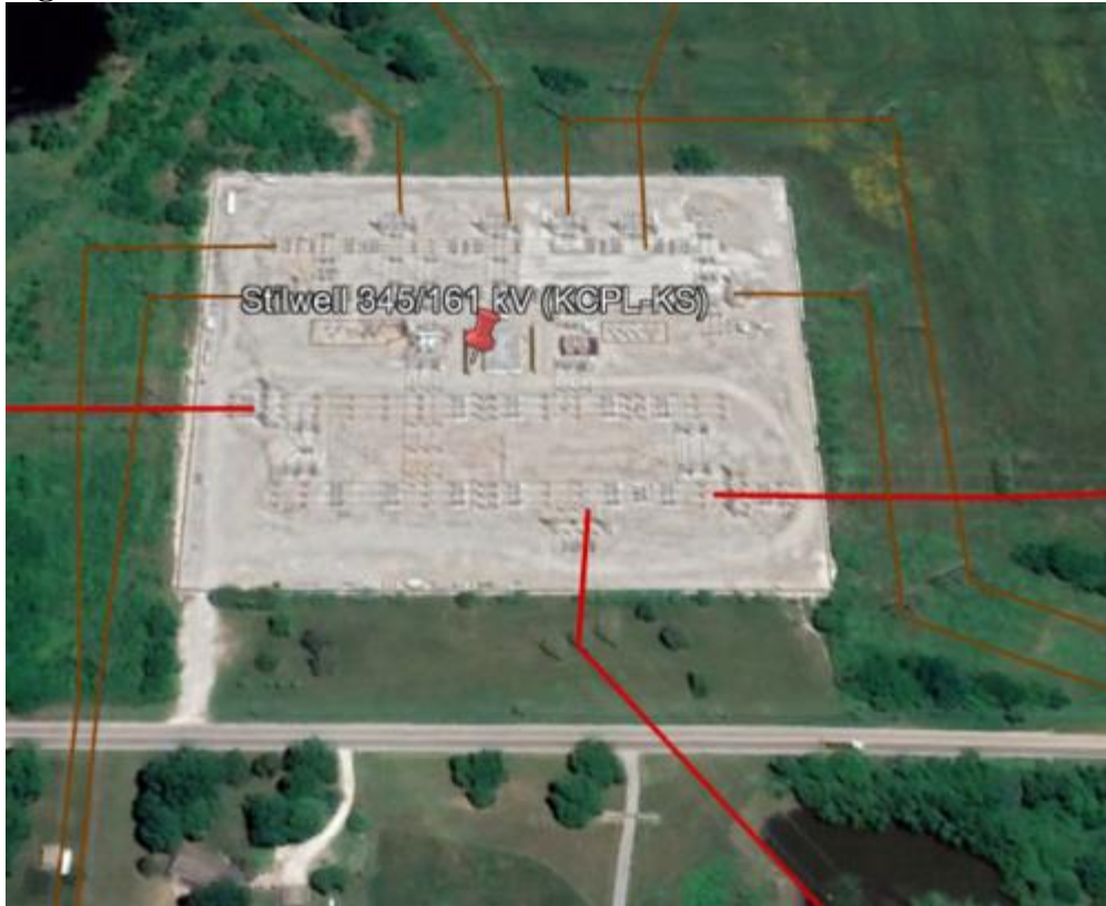
Figure 28 – Stilwell 345 kV substation
